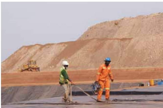
Construction of second tailings facility
